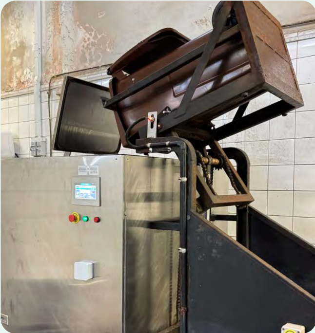
▲ Food waste bin, distinct from other bin types, is being emptied into the food waste treatment system.
