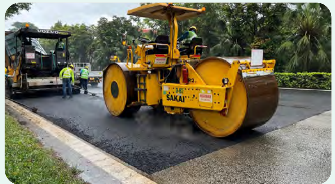
▲ New road mix for expressway (top right) on trial at PIE near Yunan Garden (bottom right).
