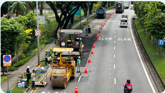
▲ New road mix for arterial roads (top left) on trial at West Coast Highway (bottom left).
