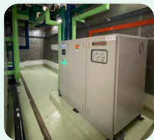
TTSH's Mini-Chiller Heat Recovery System helps to save energy by replacing energy-consuming electric heaters with heat generated from the mini chiller.
