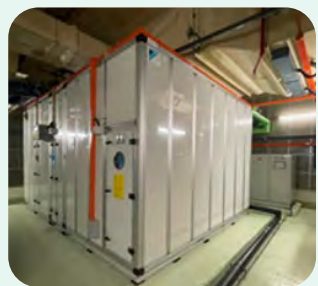
TTSH's Mini-Chiller Heat Recovery System helps to save energy by replacing energy-consuming electric heaters with heat generated from the mini chiller.
