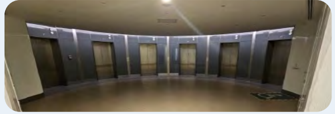
▲ Dimmed lift lobbies after office hours.
