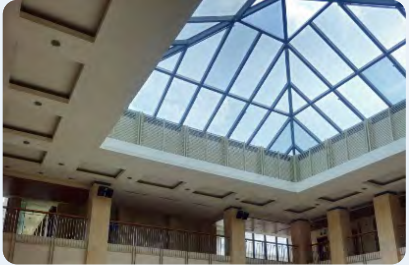
Pyramid skylight at MFA Atrium reduces the need for artificial lighting.
